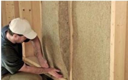
3 Make sure there is no gap between the connecting joint of two panels to avoid any loss or air infiltration.
